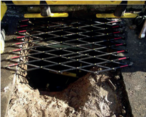
The trellis is pulled out to form a safety cover over the trench; the trellis can be clipped down for extra stability.
